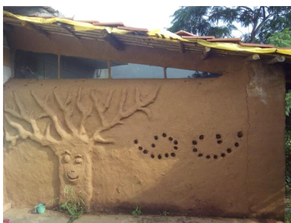
Cob-walled extension of a room
